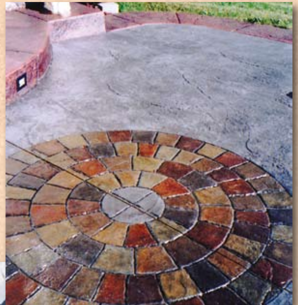
Ashlar Slate design in Sandstone Integral color and highlighted with Brick Red highlighting color.
